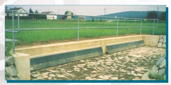
Typical installation: The ACU-FLAP Check Elements at overflow structure.
